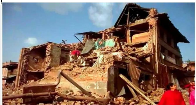
Building damaged during Earthquake of April 28, 2023 in Bajuar District
