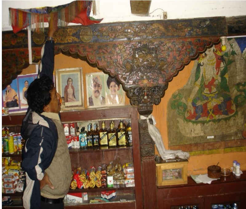
Figure 6. Wooden Post with carved bracket supporting Beam
