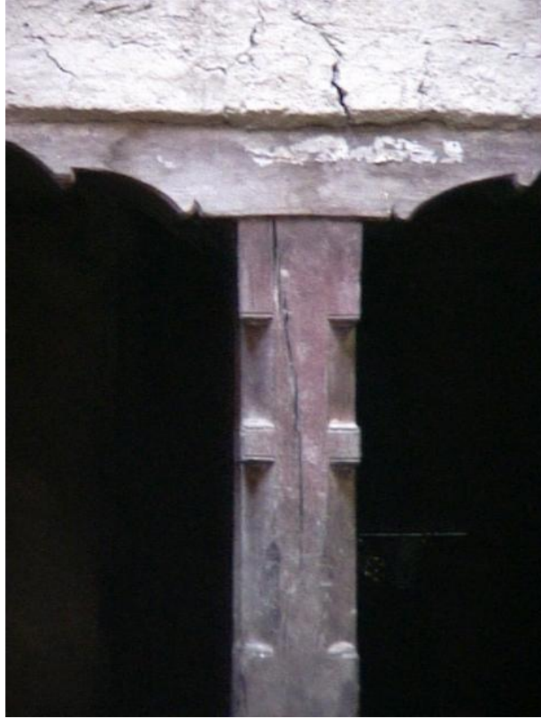
Figure 27. Detail of timber post in the dalan structure.
