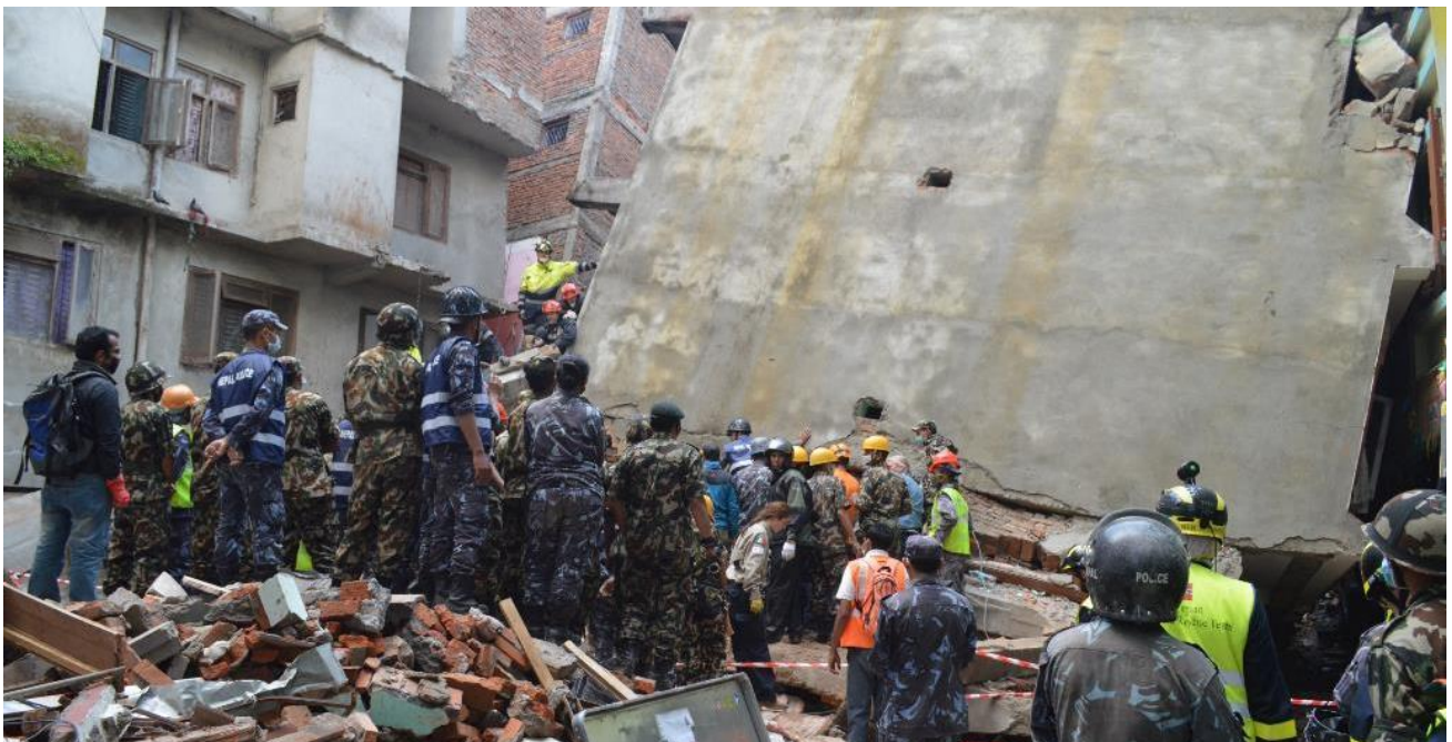
Figure 4. Some pictures of Building Damages in Kathmandu during Earthquake of April 2015
