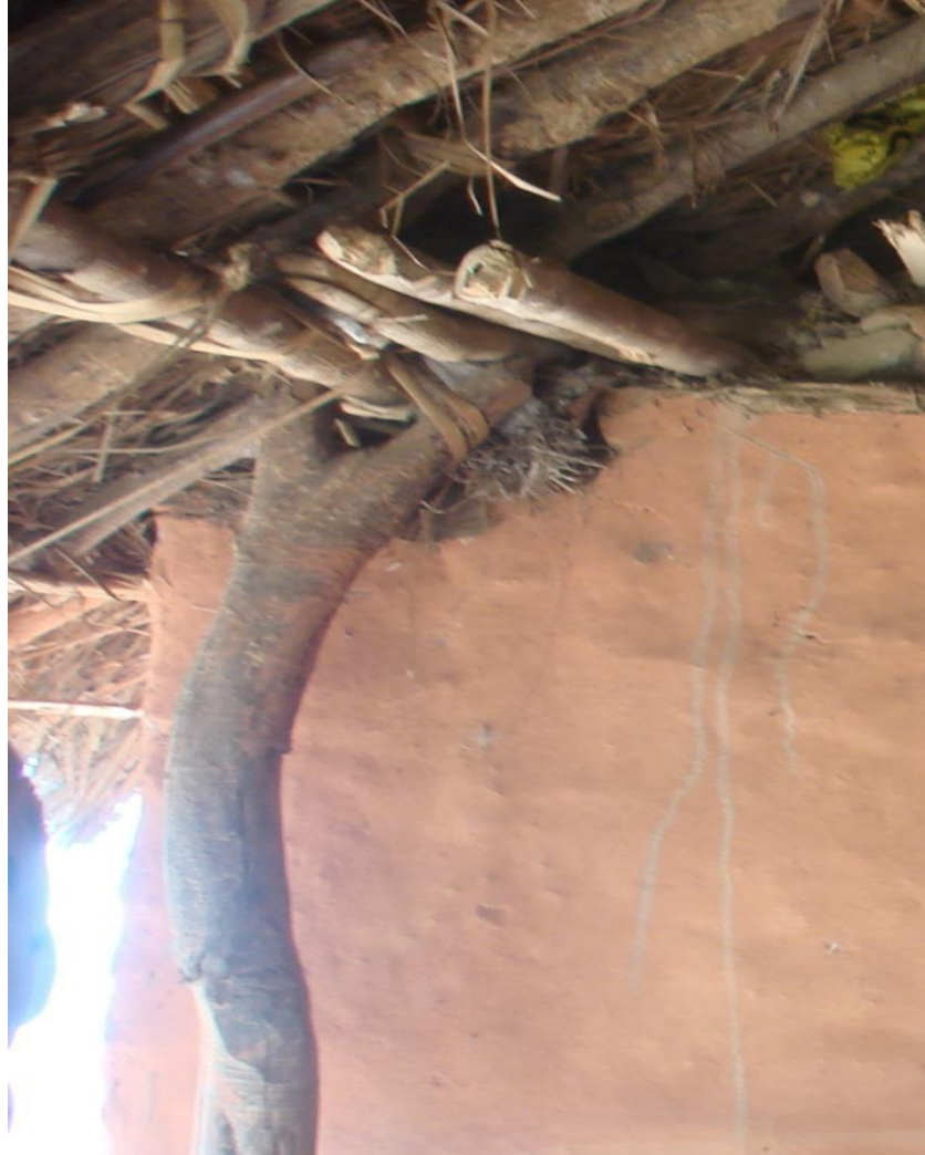
Figure 16. Detail of Pillar and Rafter Joint
