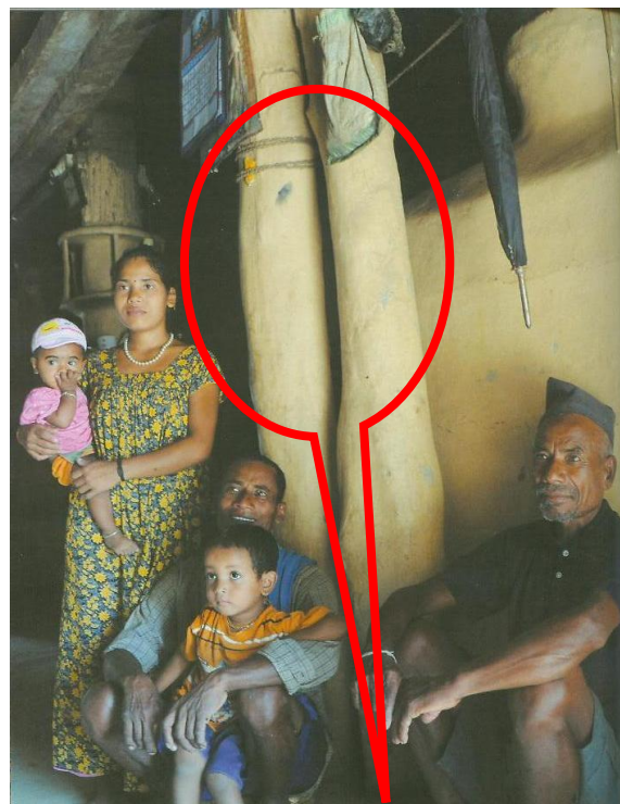
Figure 22. Two timber posts
